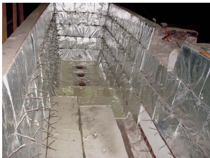
Fig. 3: Installation of PROMALIGHT®-1000 in a tundish
