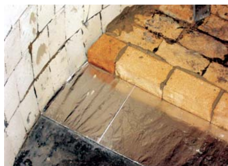
Fig. 2: Insulation of steel casting ladle
