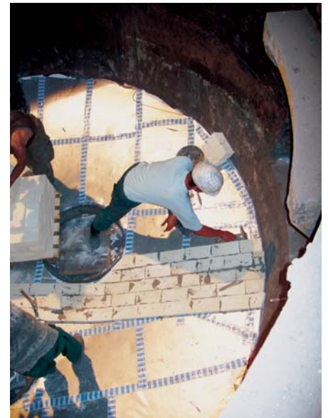
Fig. 6: Installation of PROMALIGHT®-330 and PROMATON® in an electric arc furnace
